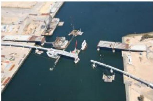
**Figure 3:** Aerial shot of the SA Port River Expressway Road and Rail Bridges in 2007, with two elevated 1000m bridges constructed for a total cost of \$178m
